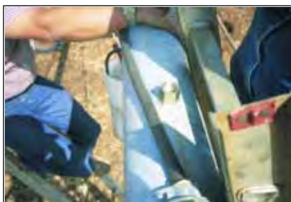
Figure 15. Swedge coupler installed.
