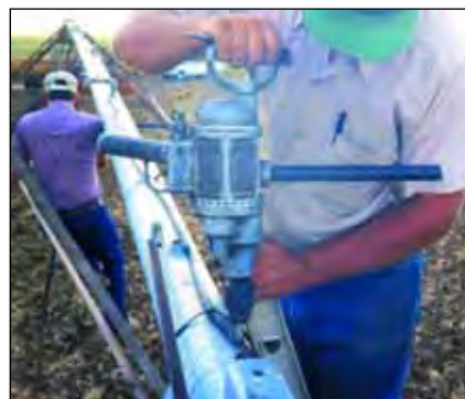
Figure 13. Drilling for swedge coupler.
