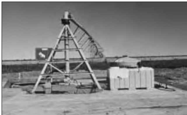
Figure 7. Center pivot sprinkler system.
