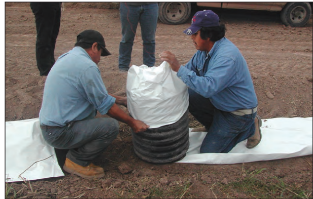
Figure 5a. Connecting two rolls of poly-pipe.
