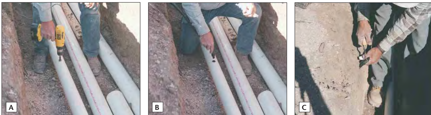
Figure 9. Drilling the manifold (A), inserting the grommet and the PVC hose (B), and connecting the PVC hose to the drip tape (C).
