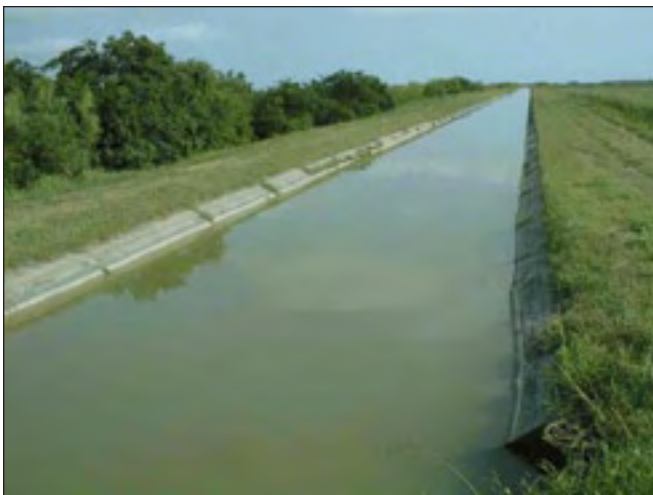
Fig. 2. Water canal lined with concrete in the Lower Rio Grande Valley.
