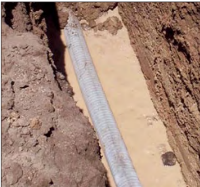
Fig. 4. Subsurface drainage used to control high water tables in the Lower Rio Grande Valley.
