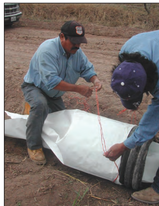
Figure 5b. Using a corrugated PVC pipe to connect two rolls of poly-pipe.
