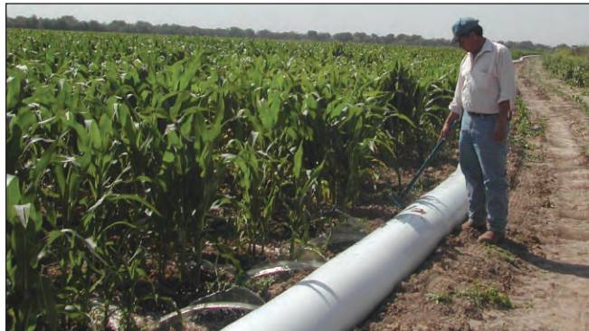
Figure 7. Using poly-pipe hole puncher.
