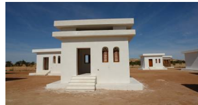
(a). Room with double roof
