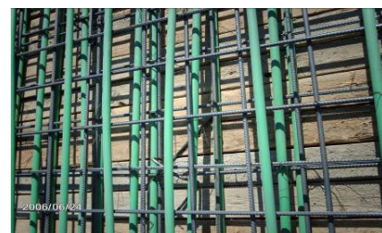
(d). Active concrete roof structure Figure 2. Photo for Test Rooms in Toshky Region.
