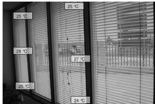
Figure 12. Surface temperature spot measurement at the façade at 2 pm
