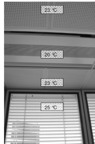
Figure 13. Surface temperature spot measurement at the ceiling at 2 pm
