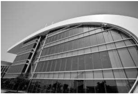
Figure 1. South Façade Office Building
