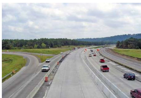
I-40 at Burns Park
