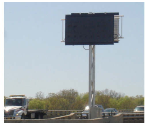
Figure 9.1 – Variable Message Sign Deployment along I-630
