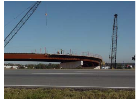
Warden Road/ Landers Road Fly-Over McCain Blvd at Hwy. 67
