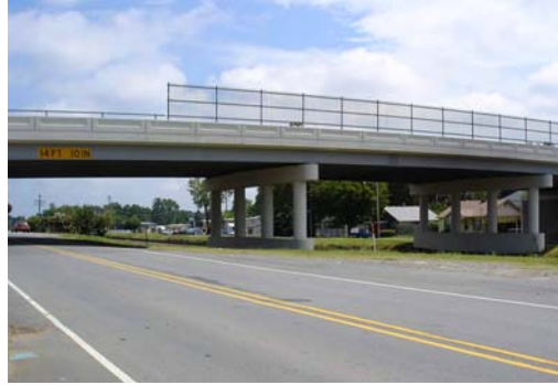
Main Street Overpass, Jacksonville
