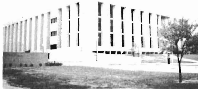
Figure 6: Example Building - The Zachry Engineering Center. One of the first buildings to participate in the LoanSTAR Program was the Zachry Engineering Center on the Texas A&M Campus. It covers an area of approximately 324,000 square foot and contains classrooms, offices and laboratories.
