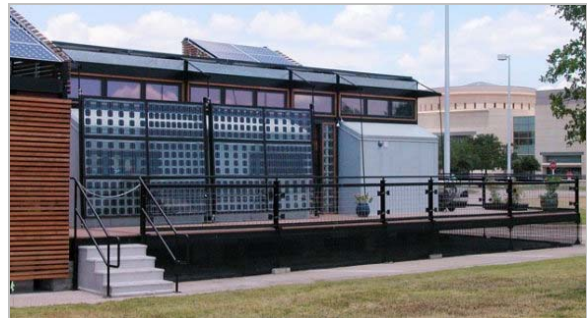
Figure 37. TAMU groHome Reassembled at the George Bush Presidential Library, Texas A&M University.
