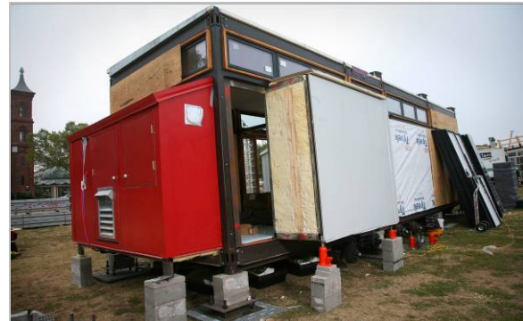
Figure 21. Installation of the groWalls.
