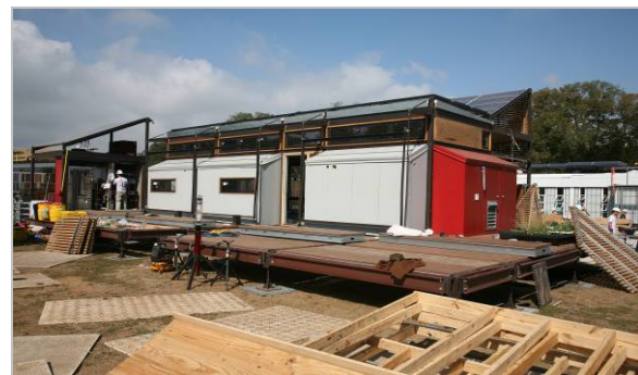
Figure 23. Installation of the Deck.
