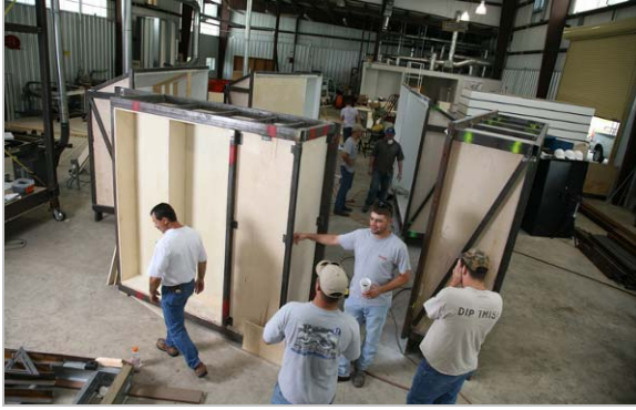
Figure 19. Construction of groWalls.
