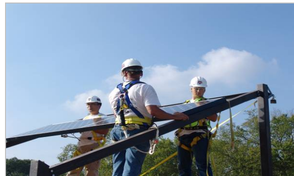
Figure 22. Installation of the PV Panels.
