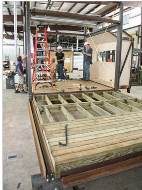
Figure 18. Construction of the Main Core.
