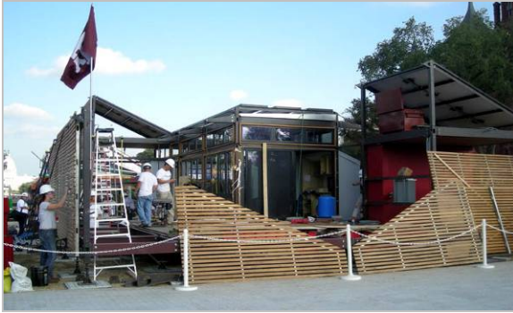
Figure 24. Rainscreen Modules to be Installed.
