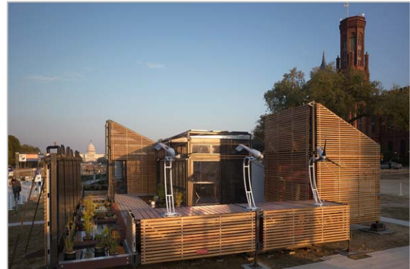
Figure 1. TAMU Solar House at the National Mall.
