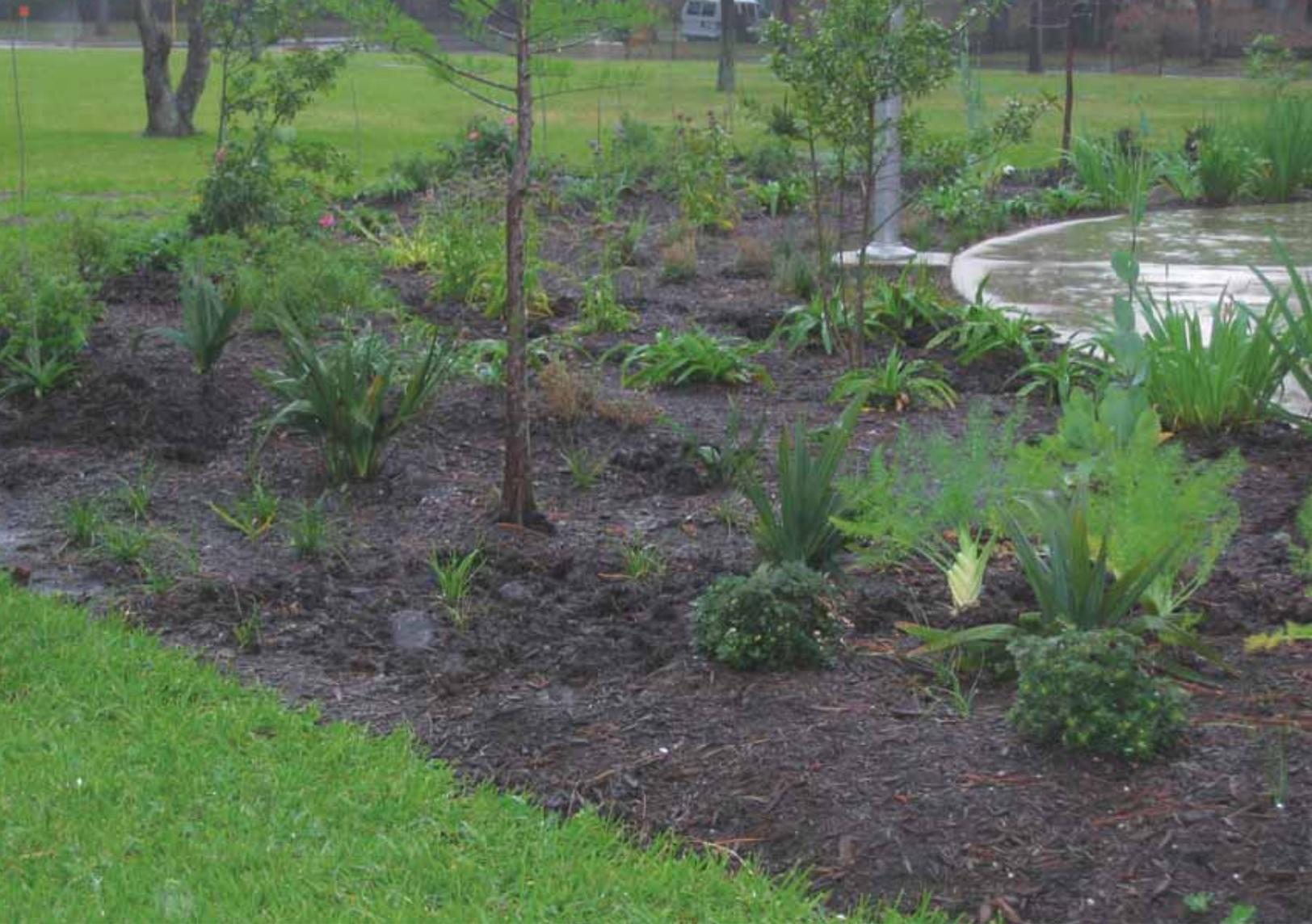
The program's Web site explains that rain gardens are made from a shallow depression in the landscape at least 10 feet from a building. The sod is removed and excavated to create a shallow, bowl-like area. Compost and sharp sand is added to the soil and planted with a mixture of native or non-invasive adapted trees, shrubs, grasses and flowers that can tolerate temporary wet conditions. A layer of mulch prevents weed growth and aids in filtration.
