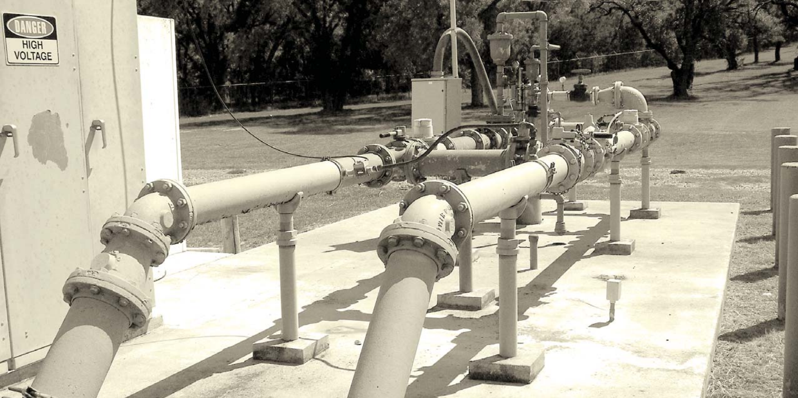
The City of Kerrville has stored excess Guadalupe River water in its ASR system since 1990. The city currently has two ASR wells. Photo by Grant Terry, city of Kerrville.
