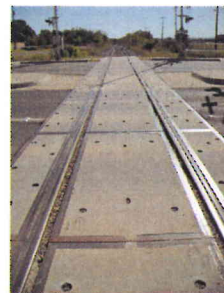
Southwest Blvd: 917 525 E – GOOD
