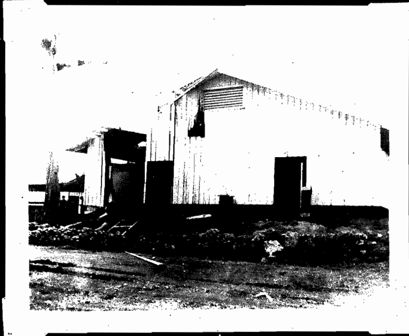
Exterior Damage - E.M. Mess Hall
