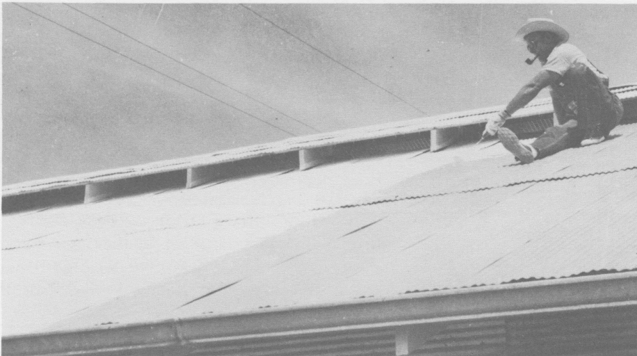
Figure 25. White roofs reflect heat, thus reducing the inside temperature of the building. This can be accomplished by painting or white washing.
