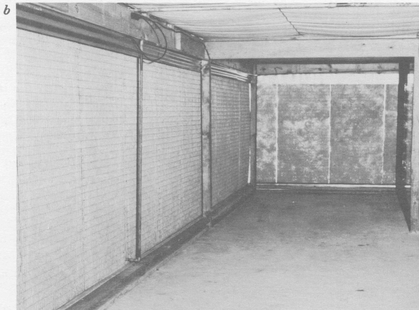
Figure 24. Pad and fan cooling systems have been reported to reduce the internal temperature of the laying house 10 degrees F. below the outside temperature. Fans are located on the opposite ends of houses from pads. (a) outside view (b) inside view (c) fan arrangement.
