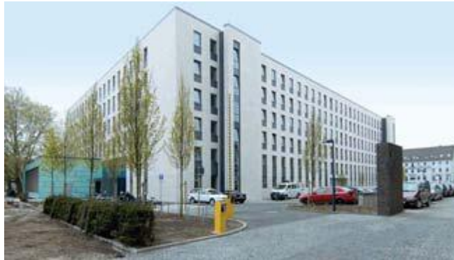
Figure 3.20 Neues Regionshaus Hannover Building
