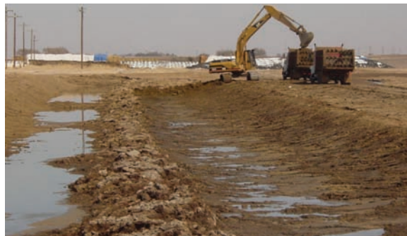
Figure 3. Gravitational solids separation basin during clean out. The water enters the basin in the foreground and slows to allow solids to separate from the water, which continues to flow through the basin and to the lagoon.
