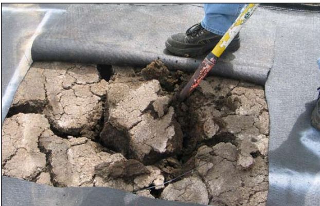
Figure 5: Residual solids in dewatered Geotube®.
