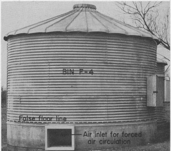
Figure 19. A type of construction for a false floor in a round steel bin.
