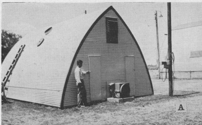
Figure 2. These steel buildings were used for drying and storage tests. A. This 16 x 28-foot building was equipped with a fan and air distribution system for drying and aerating grain. B. Two 50,000-pound capacity bins were constructed in this 32 x 60-foot steel building.
