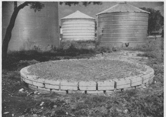
Figure 8. Foundations made by setting a ring of concrete blocks and filling the inside with well-tamped earth were used for most of the round steel bins.
