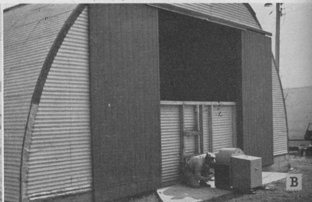
Figure 2. These steel buildings were used for drying and storage tests. A. This 16 x 28-foot building was equipped with a fan and air distribution system for drying and aerating grain. B. Two 50,000-pound capacity bins were constructed in this 32 x 60-foot steel building.
