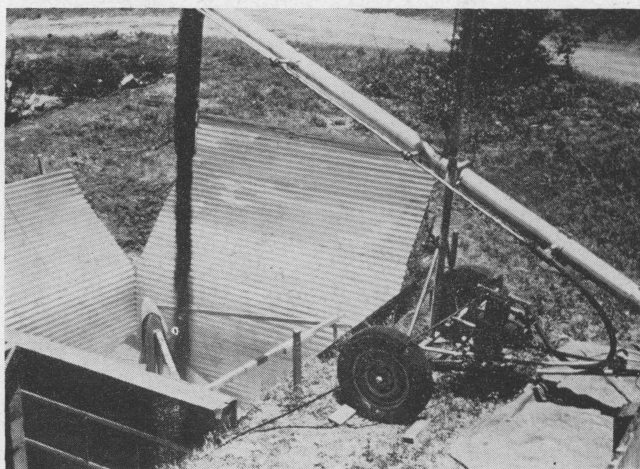
Figure 6. Underground pits were used to determine the practicability of this type of storage in South Texas.
