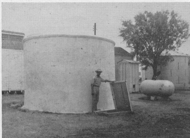
Figure 3. This 56,000-pound capacity cement plaster bin was equipped with a screw conveyor in the bin floor to facilitate unloading. A removable cover, shown in raised position, was used to keep water out of the unloading pit. To prevent spoilage of grain in the surface layer, it later was necessary to install a revolving head ventilator in the bin roof.
