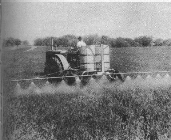
Figure 15. A properly equipped boom-type sprayer gives the most accurate spray placement and consistent weed kills. (Photo courtesy of Century Engineering Corporation, Cedar Rapids, Iowa.)
