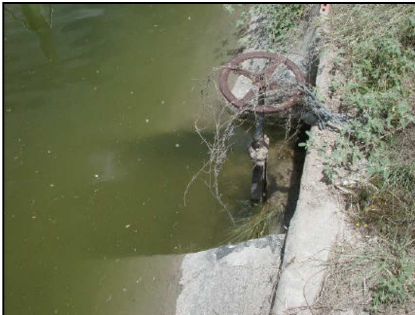
Figure 6. Turnout gate located in test segment 16HC1.
