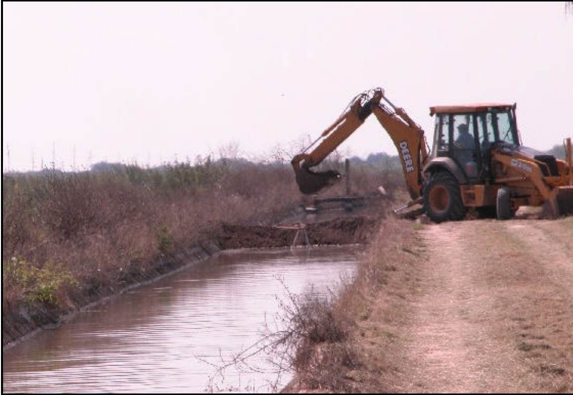
Figure 4. Photograph of district's backhoe constructing earthen dam for a ponding test.
