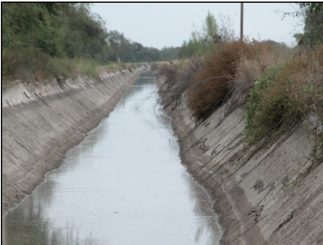
Figure 1. Photograph of test segment 16HC1 of the Main Canal B.
