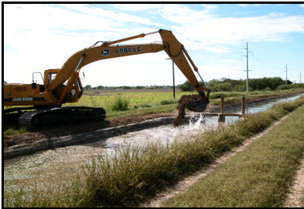
Figure 3. Photograph of district's backhoe constructing earthen dam for ponding tests.
