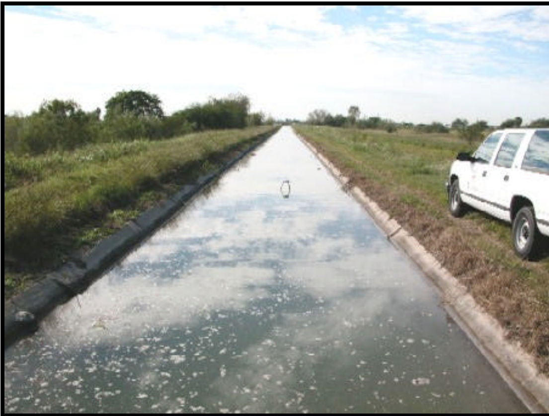
Figure 1. Photograph of test segment SJ9 of the North Alamo Main Canal.
