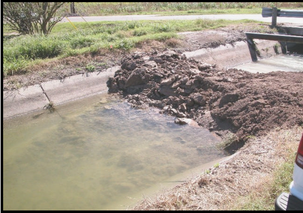
Figure 4. Close up photograph of earthen dam use to seal test segment.
