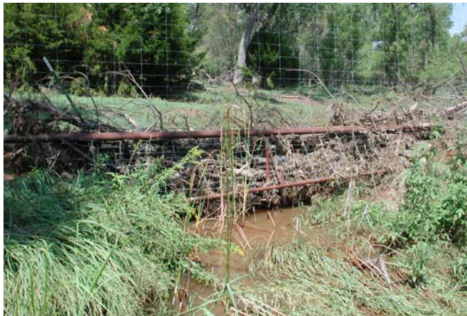
Evidence of high flow in Buck Creek
