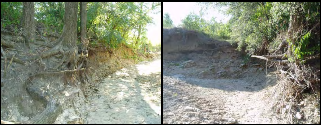
Fig. 5: Stream bank de-stabilization
