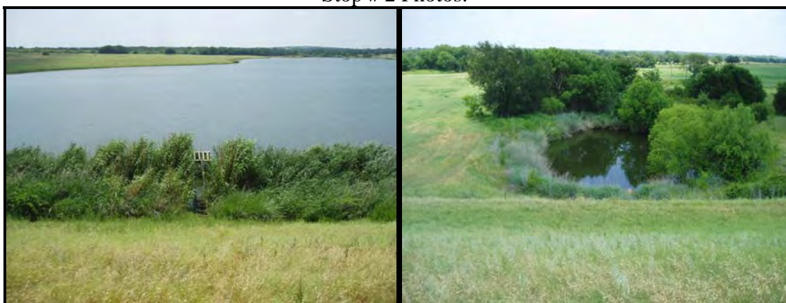
Fig. 7: Principal spillway and good cover
