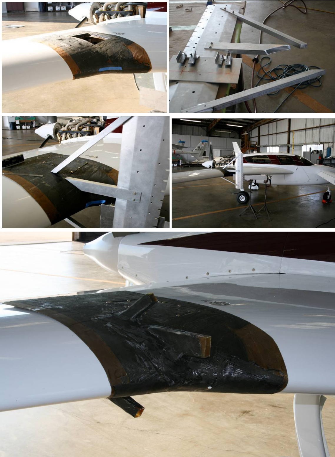
Figure A.98 Stages of Construction on the Wing Glove and Attachment to the Pressure Rake
