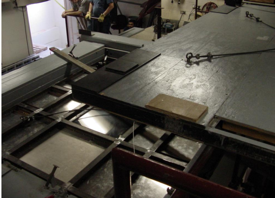
Figure B-3 Installation of the roof
