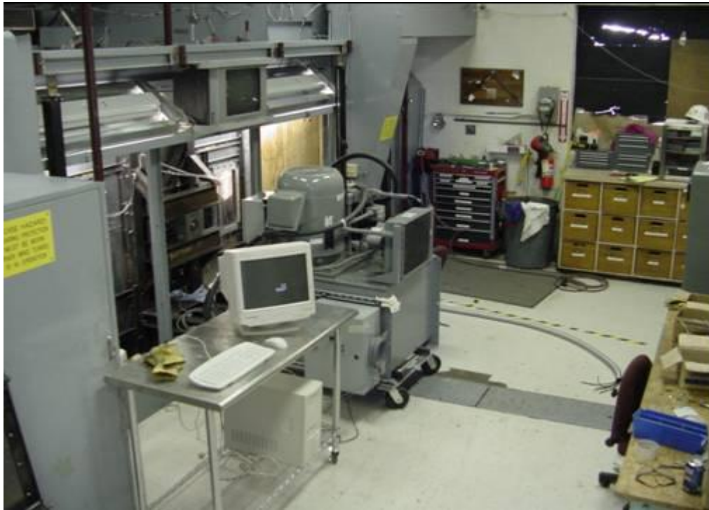
Figure 61: Image of the hydraulic actuator drive system
