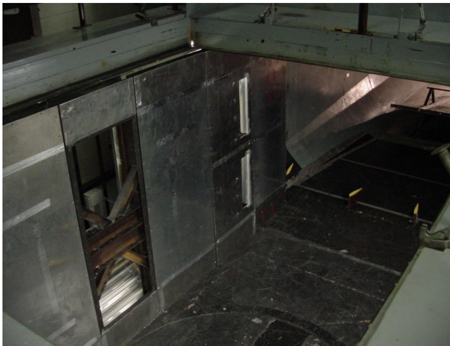
Figure B-2: Installation of the left wall
