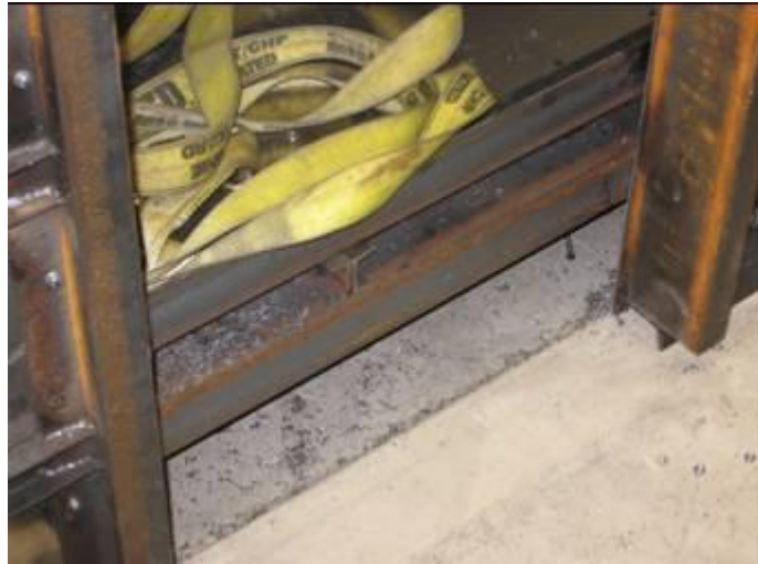
Figure 31: 3 in x 3 in C-channels bolted to the steel frame of 7 ft x 7 ft wind tunnel
