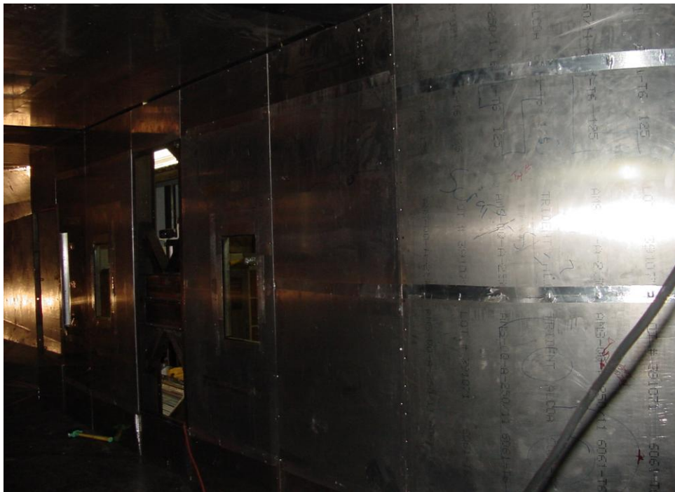
Figure B-5 Installation of left wall with the inlet section
