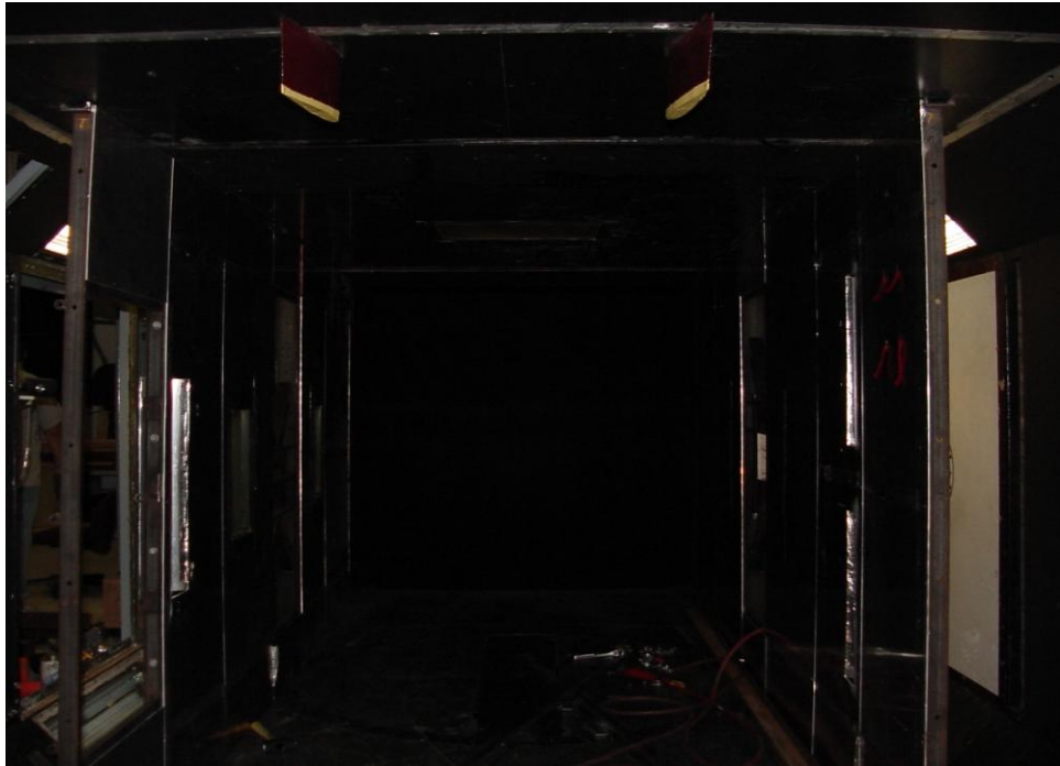
Figure B-4 Installation of side walls and roof - loosely connected
