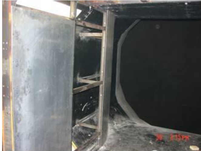
Figure 25: Steel frame of inlet screwed to the concrete
