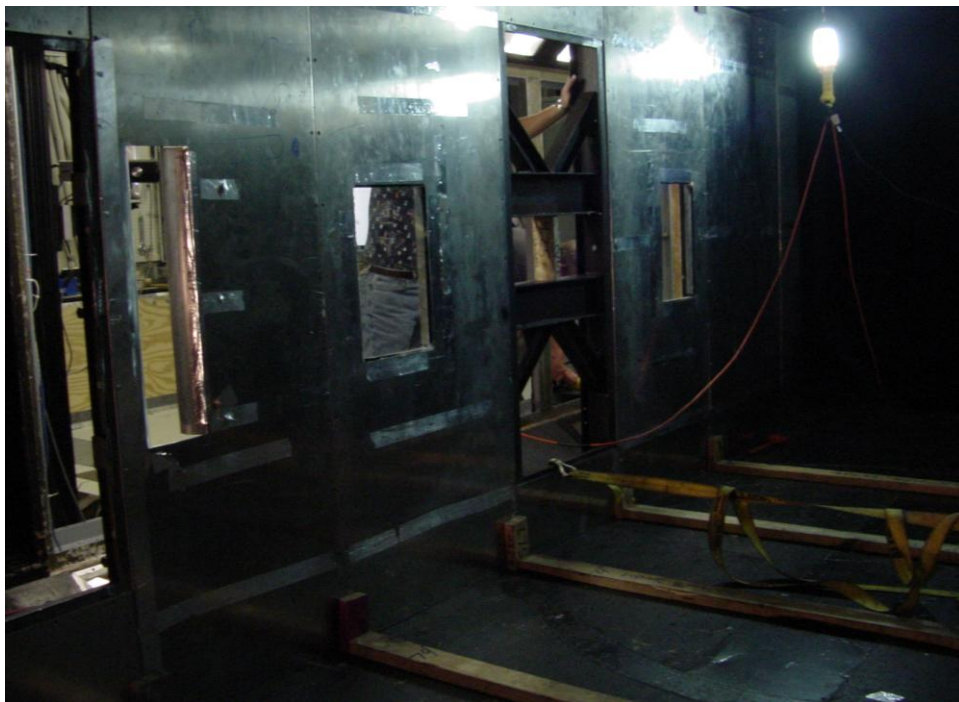
Figure B-7 Alignment of side walls with 2 by 4s
