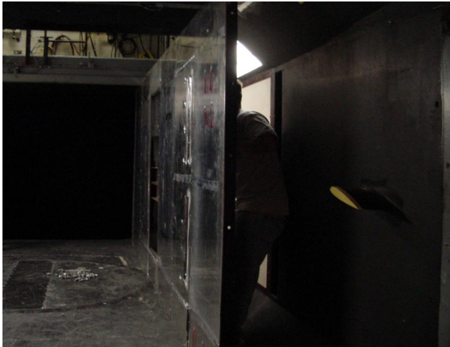
Figure B-1: Installation of the right wall
