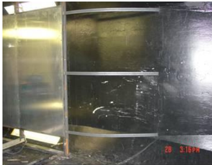
Figure 23: Curved steel frame of the inlet
