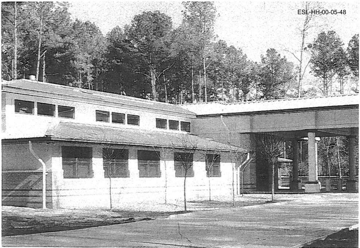
**Figure 1:** South elevation of Texas Specialist Center. Note clerestory windows for daylighting & thermal siphoning. Light colored paving reduces site ambient temperatures. Photovoltaic panels are on upper roof.
