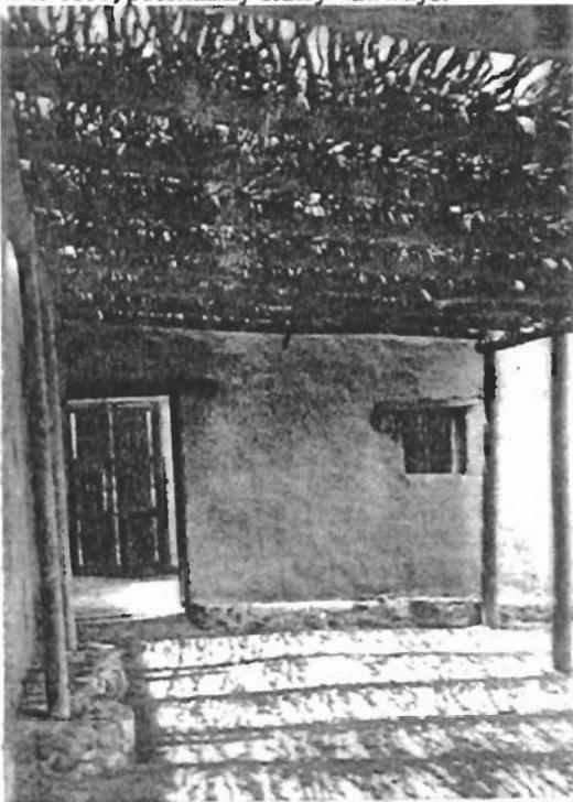
Fig. 1 Ramada at Fort Leaton, Texas
