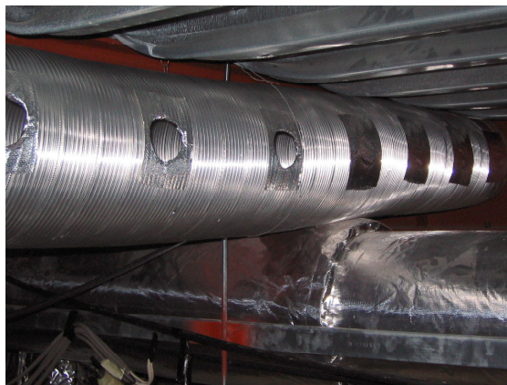
Photo 1 Header type openings installed in the ceiling space
