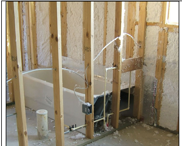
Figure 4 Draft stopping and Insulation behind tub (TWH)
