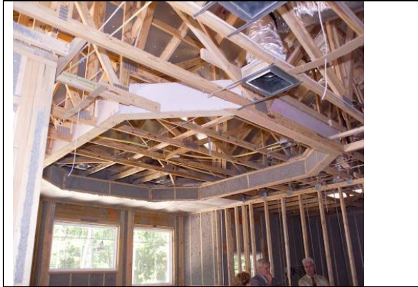
Figure 3 Solid blocking at tray ceiling framing (GWR).
