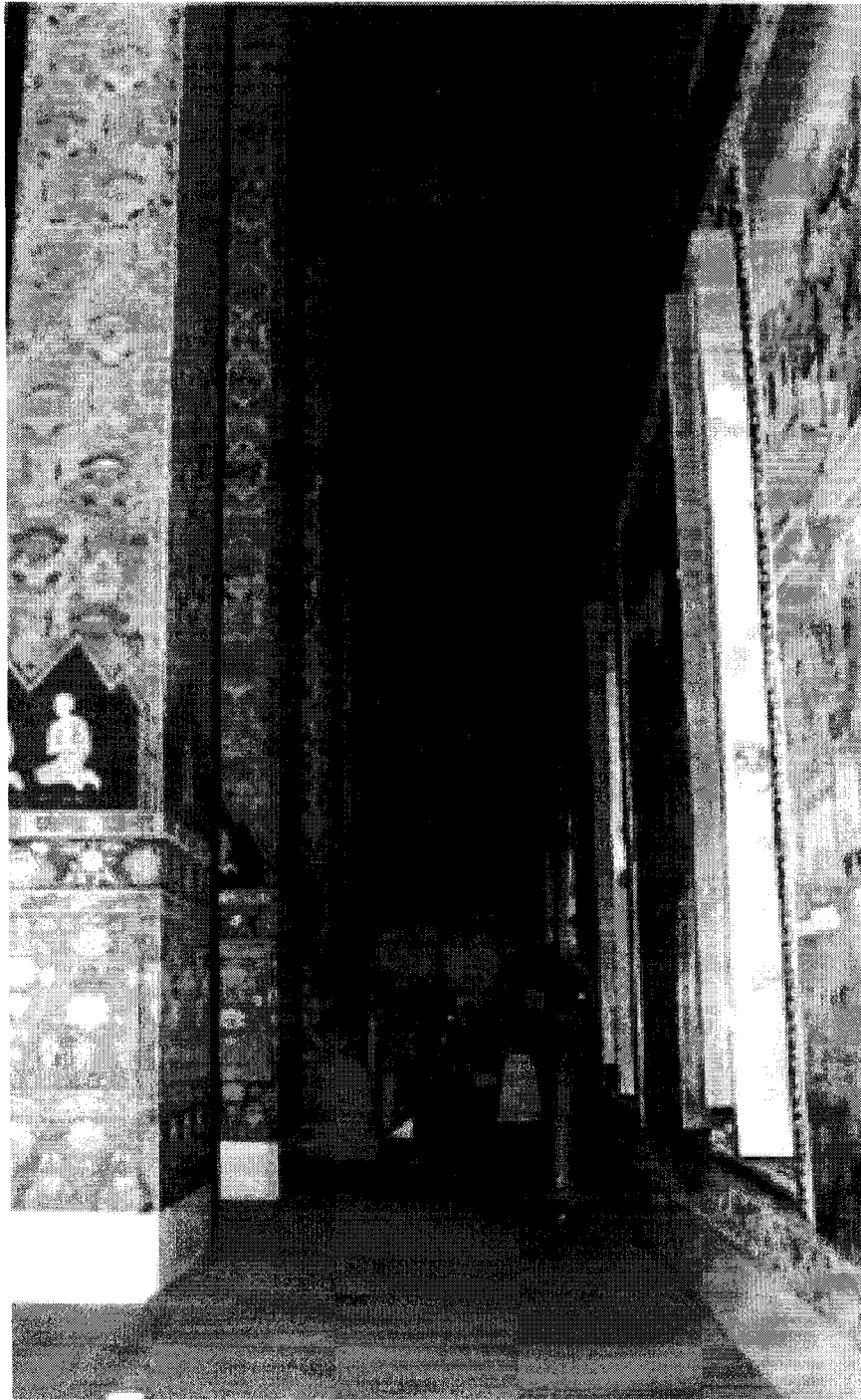
Figure A.3 Interior View of the Old Temple Showing the Interior Corridor. This picture shows that a portable fan was used to provide comfort to occupants. It was found that the indoor was dark during the day because of insufficient daylight.
