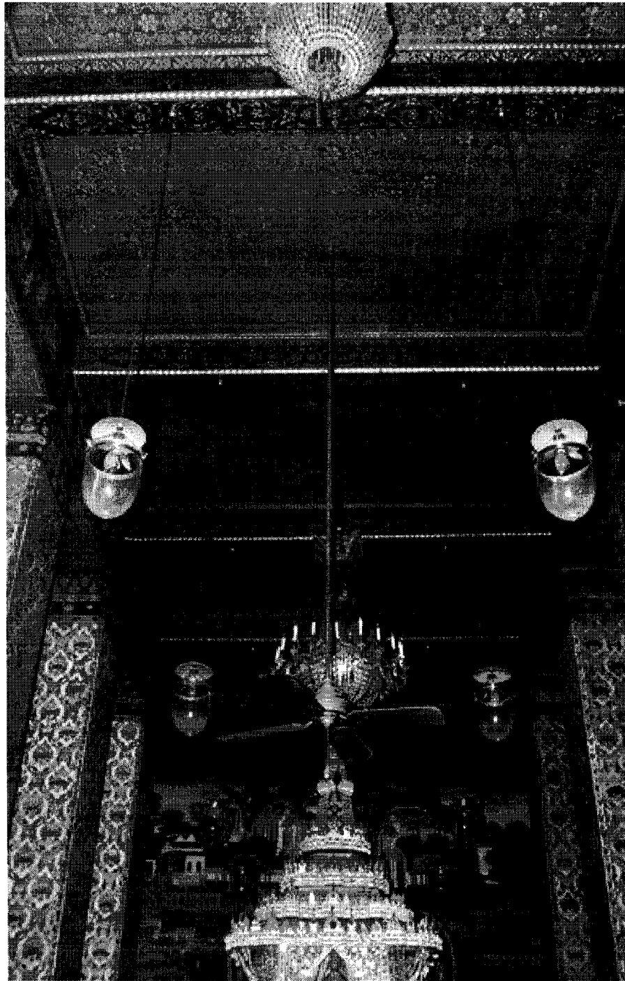
Figure A.2 Interior View of the Old Temple Showing the Wooden Ceiling, a Chandelier, Ceiling Lamps, and a Ceiling Fan. The ceiling fan and the chandelier were found to be broken. It is difficult to replace the lamps because of the height of the ceiling.
