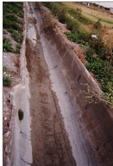
Figure 13. Improvements to canals such as this one in the Lower Rio Grande Valley will mean a net increase in available water due to lessened conveyance losses.
