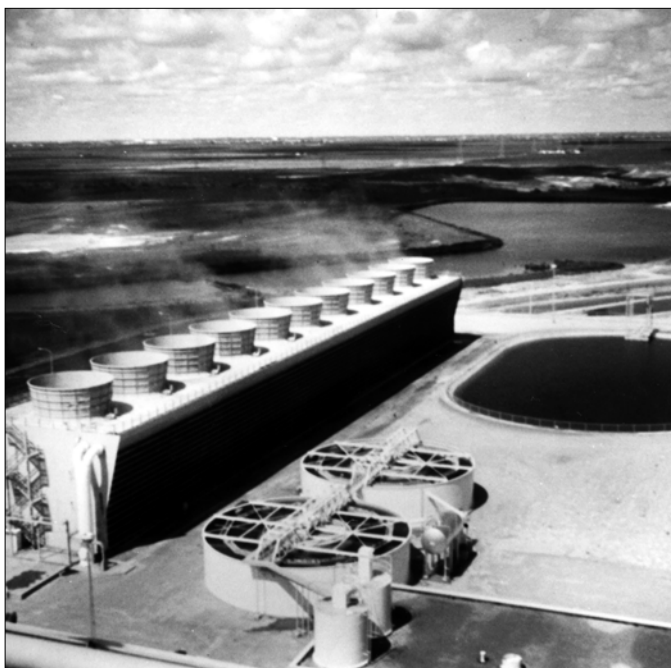
Figure 9. Southwestern Public Service in Amarillo uses treated wastewater in cooling towers at its Panhandle power plants. It sells wastewater from cooling tower operations to a farmer for forage irrigation.
