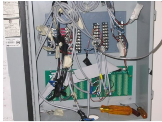
Figure 7.11 Junction box connection from different test component
