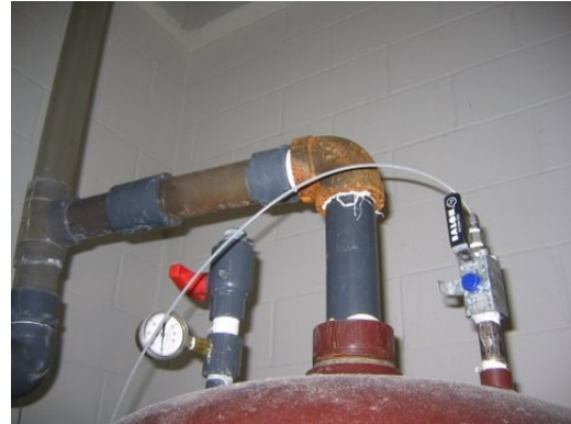
Figure 7.5 Pressure transmitter connection at the wellbore and pressure gauge to measure the wellbore pressure
