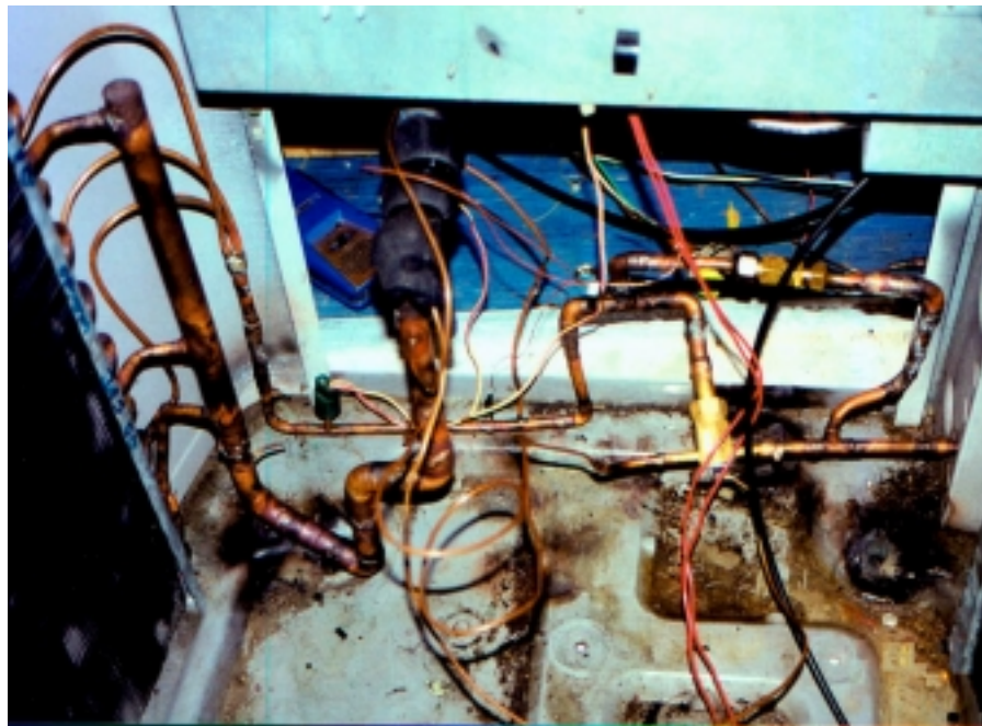
Figure 3.14 The combination of TXV and check valve inside the outdoor coil cabinet
