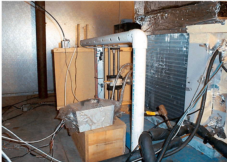
Figure 3.26 The video camera moving facility
