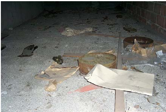
Measure 1: Insulation of the crawl roof space
