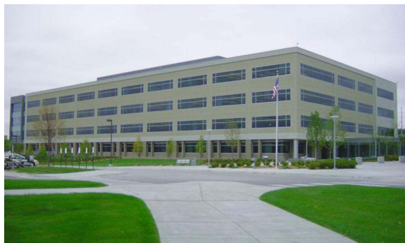
Figure 14 Case Study Building
