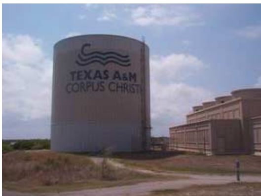
Figure 2. The thermal storage tank
