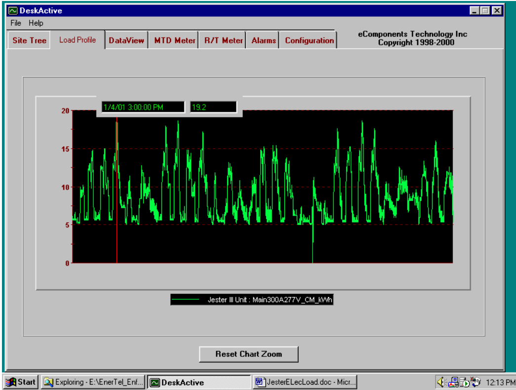
Figure 2. Screen Shot of Main Electrical Service kWh for Jester III Unit at TDCJ.
