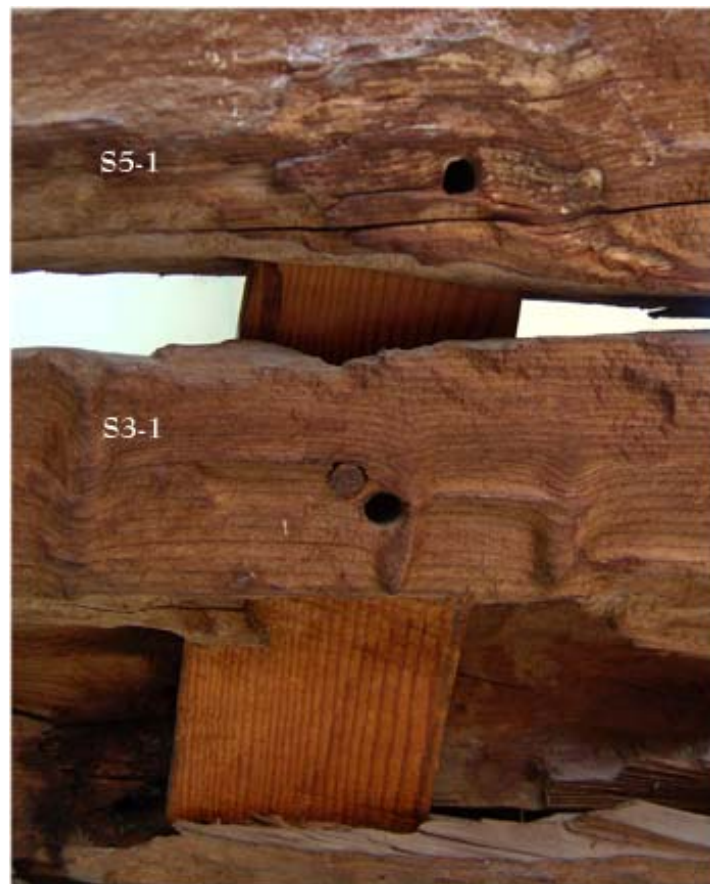
Figure 48. An ancient mortise with pegged modern tenon in GC 4926 (P. Creasman).
