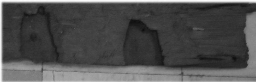
Figure 47. Exploded mortises from the underside of a deck plank - GC 4926 (P. Creasman).
