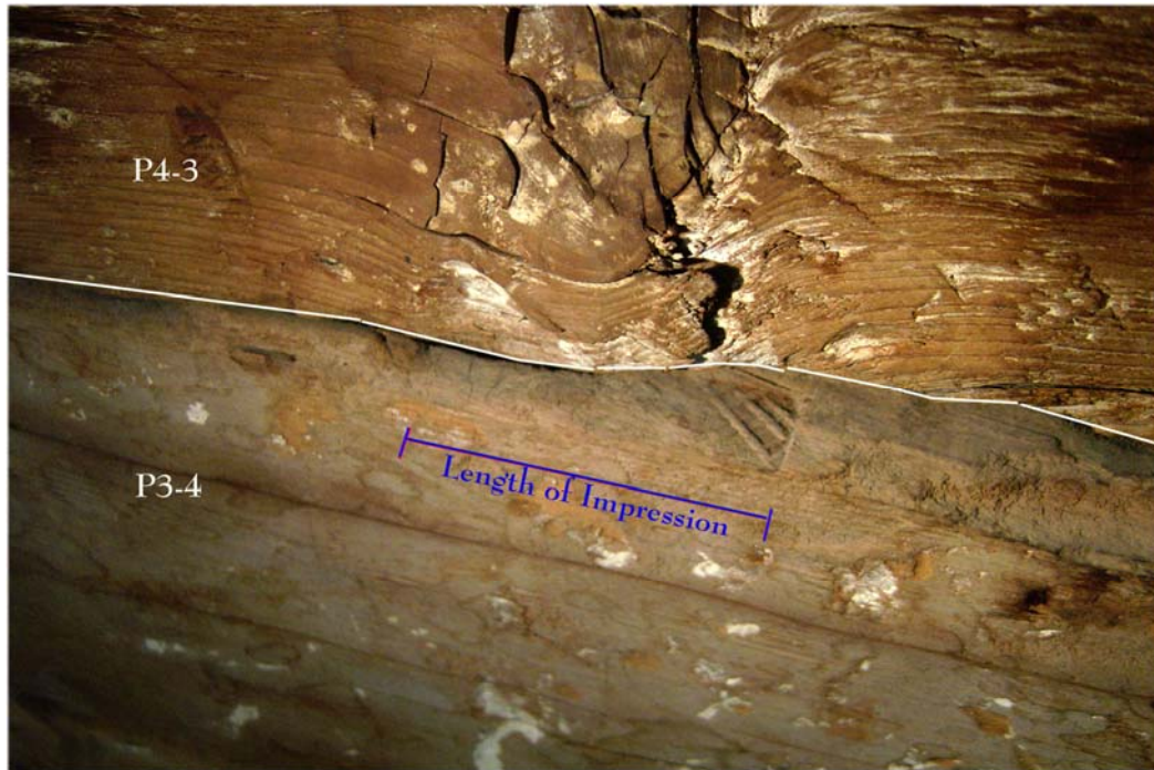
Figure 28. Close up of a cross-hatched impression at a mortise on the de Morgan boat (J. Levin).
