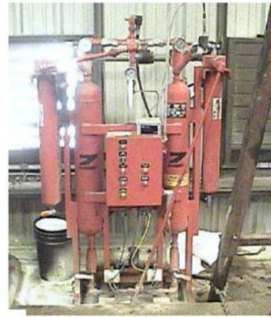
Figure 9: a) Chicago Pneumatic compressor. b) Domnick Hunter air dryer
