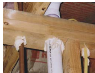
Figure 6. Sealed penetrations
