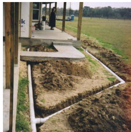
Figure 10. Manifold for rainwater collection
