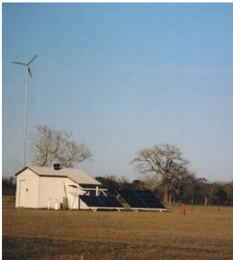
Figure 7. Hybrid PV/Wind system
