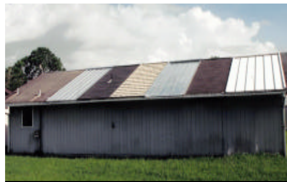
Figure 2. Flexible Roof Facility in summer 2002 configuration.
