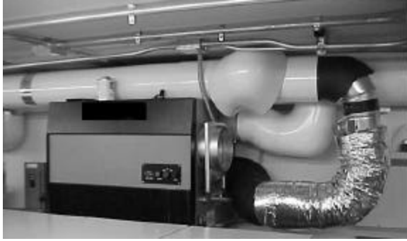
Figure 2 – Dehumidifier DH-3 during regeneration control damper installation.
