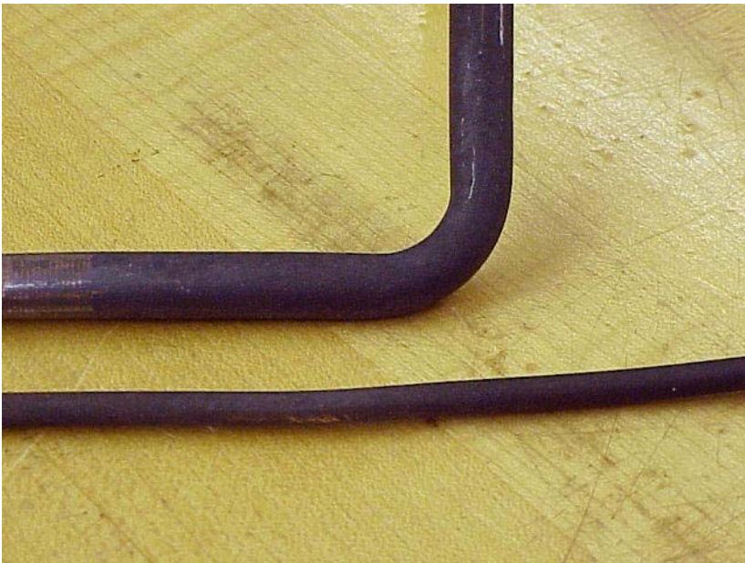
Figure 4. Appearance of sulfur attack on copper tubes.
