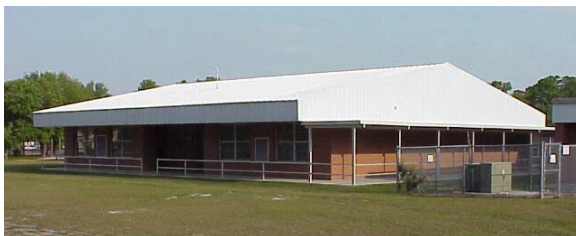
Figure 1 Typical quad classroom building
