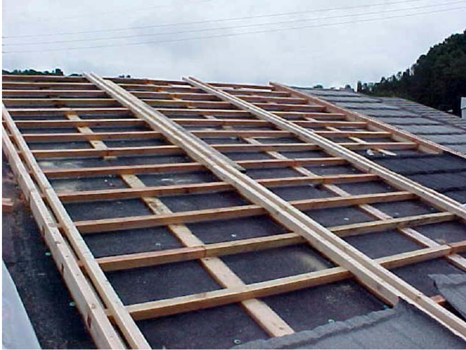
Figure 3. Roof deck construction with battens and counter-battens.
