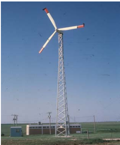
Figure 1. The Enertech Wind Turbine Installed in Randall County, Texas
