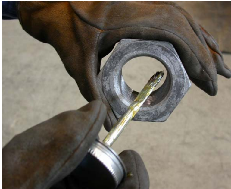
Figure 2.5 – Lubricating nut threads
