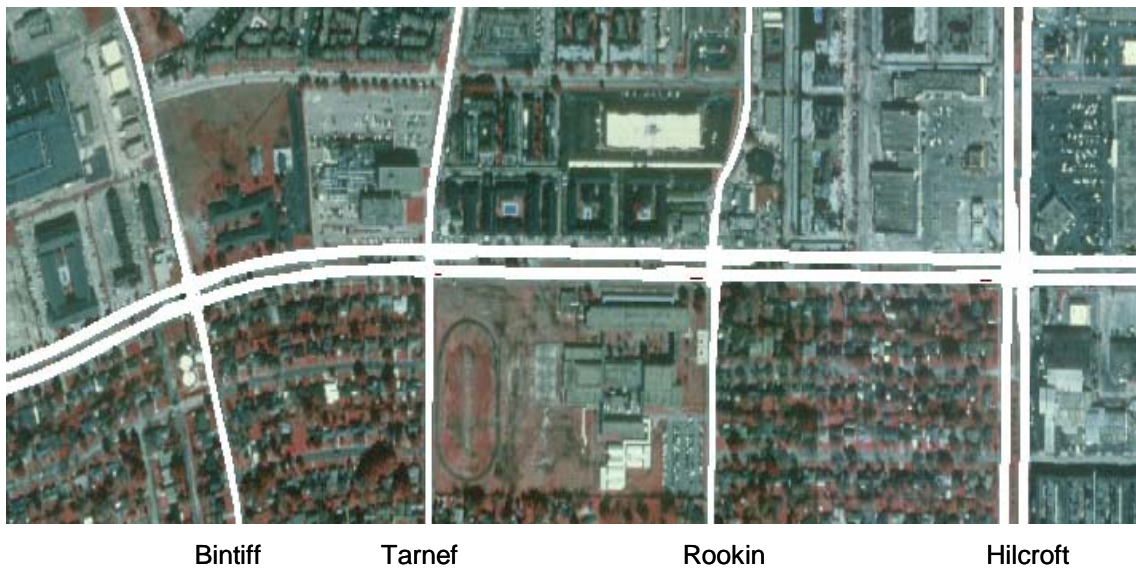
FIGURE B.3 Aerial Photo Map of the Bellaire Arterial Test Network in Houston
