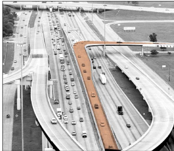
FIGURE 2.2 An access/exit T-ramp on Katy Freeway HOV lane.
