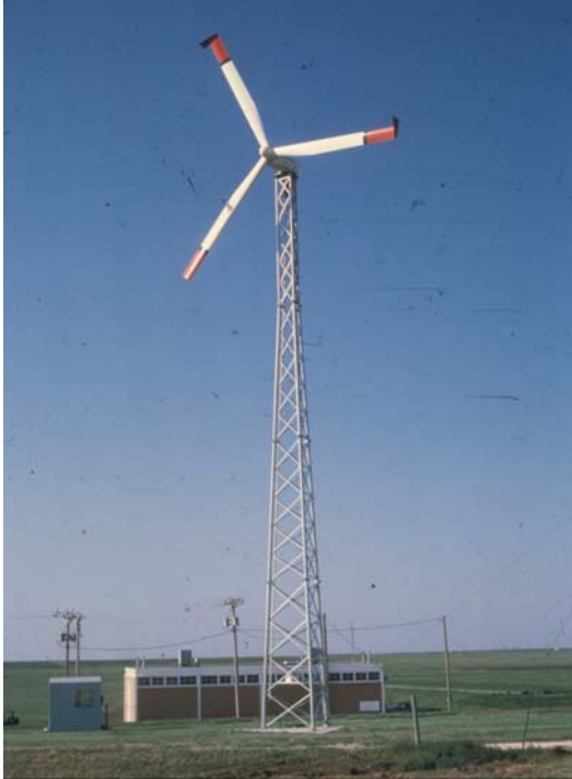
Figure 15: The Enertech Wind Turbine Installed in Randall, Texas
