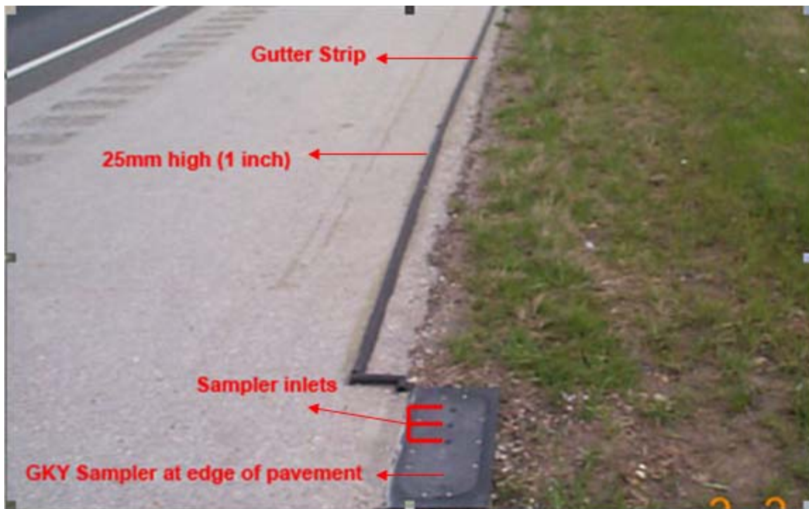
Figure 3.10. Installed sampler at the edge of pavement at College Station
