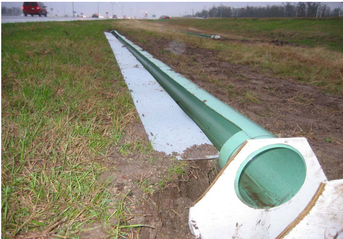
Figure 3.6. Design of a collection pipe
