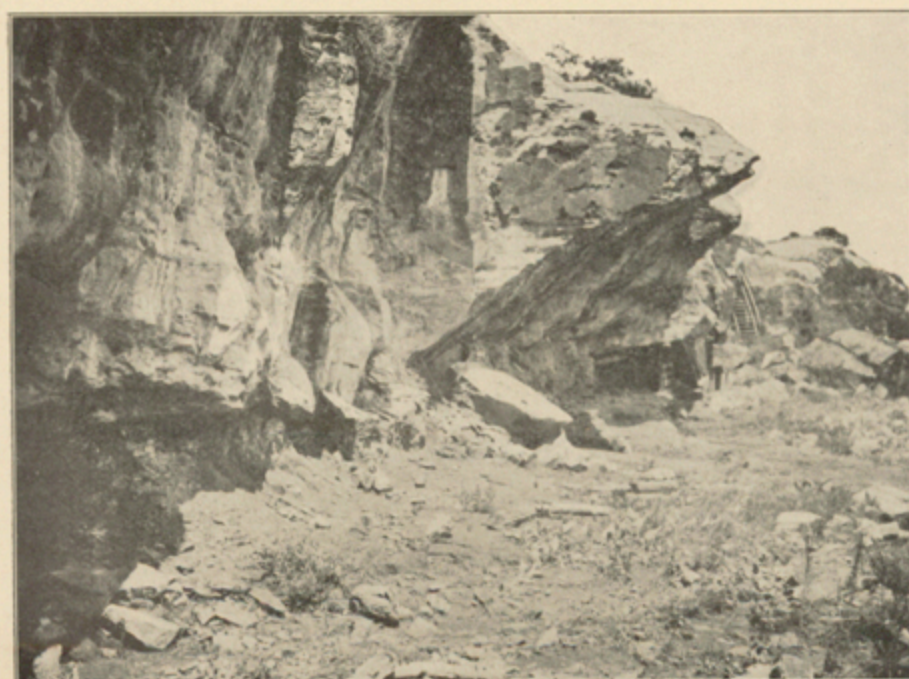
PLATE XI.—OLD FIRE-CLAY WORKINGS IN DARK SHALE AT THE TOP OF THE PURGATOIRE FORMATION AND OVERLYING MASSIVE DAKOTA SANDSTONE, 2 MILES NORTHEAST OF THATCHER.
