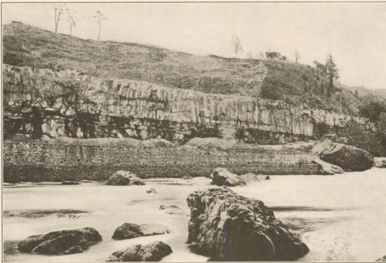
FIG. 29.—CONFORMABLE CONTACT OF BASALT OF THE FIRST WATCHUNG SHEET ON NEWARK SANDSTONE, BELOW FALLS OF THE PASSAIC, PATERSON, N. J. The sandstone forms the base of the section immediately above the retaining wall and is overlain by massive-bedded basalt capped by finely columnar basalt.
